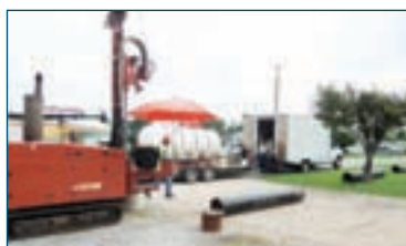
Drilling vertical holes for a CTHDD project
