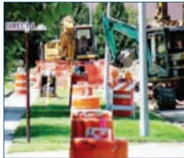
Trenchless Flowline work site in Baton Rouge, Louisiana
